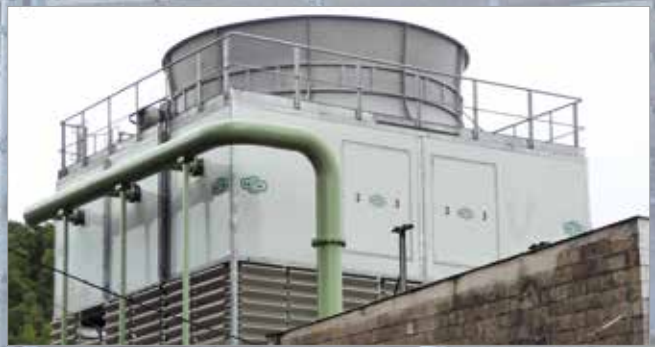
Plant after the replacement with MITA modules
