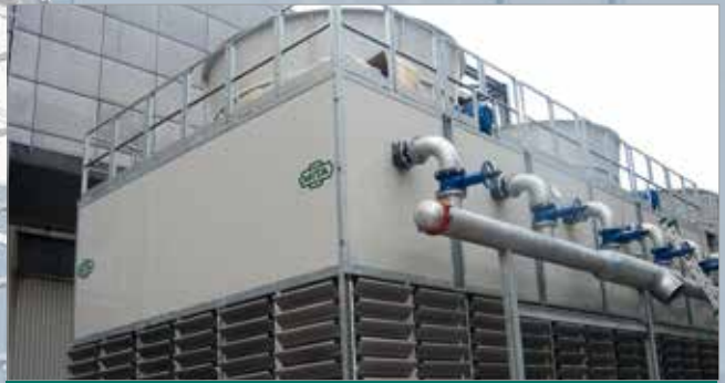
Plant after the replacement with MITA modules
