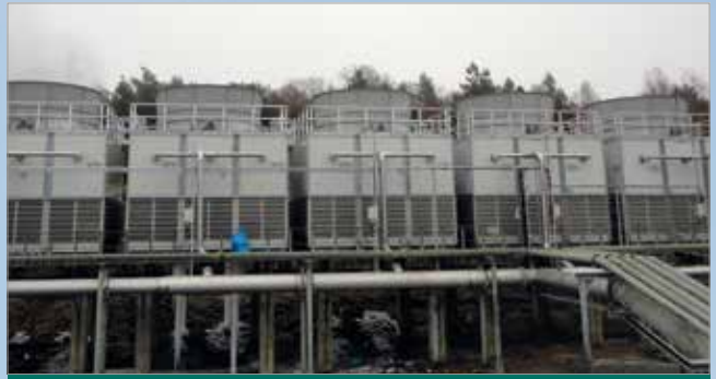
Plant after the replacement with MITA modules
