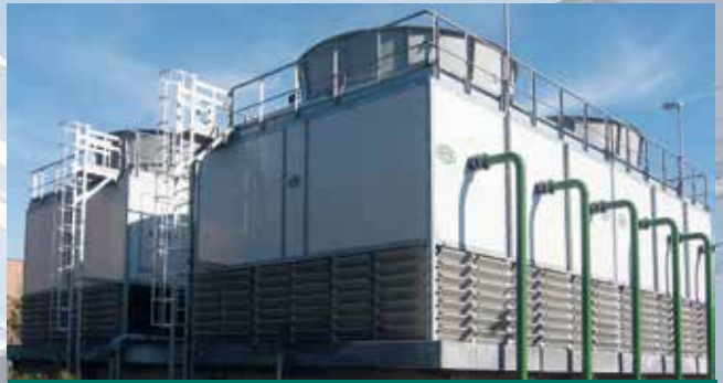
Plant after the replacement with MITA modules
